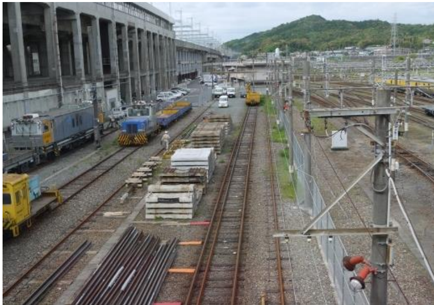
Shinkansen maintenance yard
