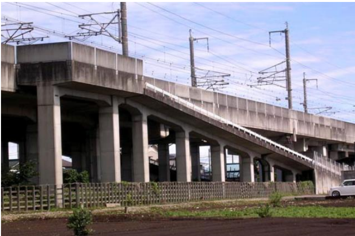
One ramp in every 5-7km as a guide (in the case of Hokuriku Shinkansen between Kanazawa and Turuga)
