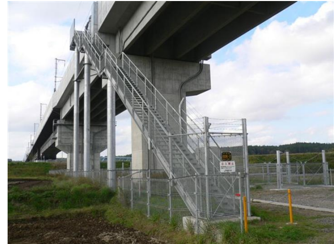
One staircase in every 1.5-3km as a guide (in the case of Hokuriku Shinkansen between Kanazawa and Tsuruga)
